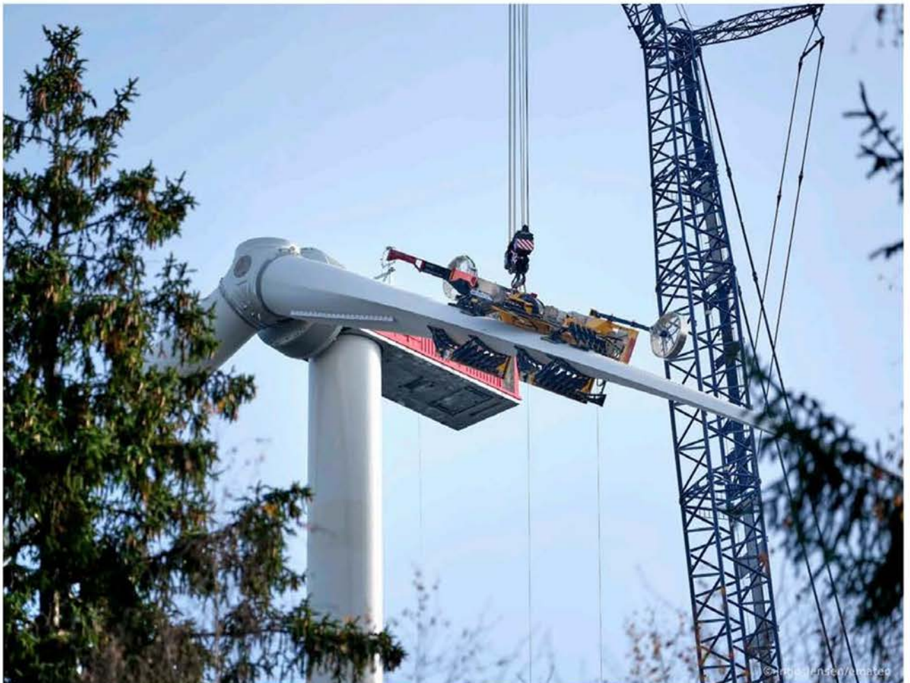
The RBC-D yoke from ematec at the wind farm Röschenwald
