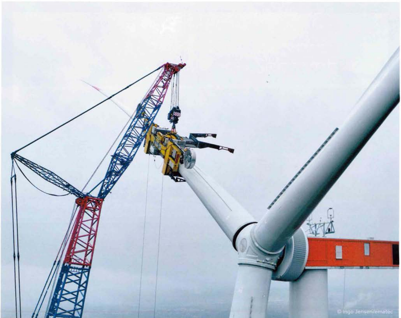
The RBC-D from ematec enables rotor blade installation at a wide range of angles within \pm 30 degrees
