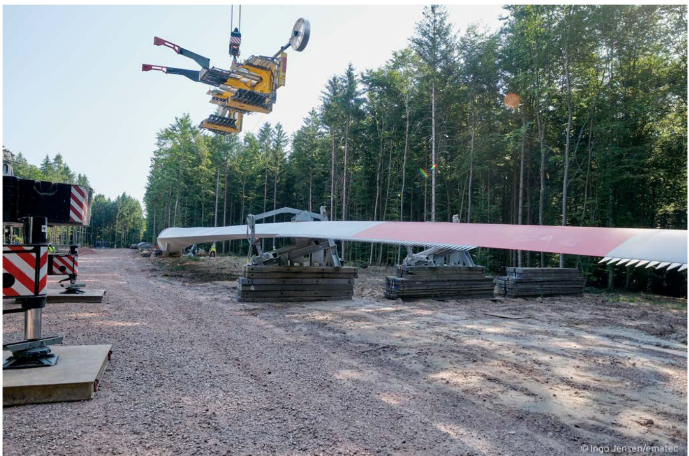
Onsite, the RBC-D and APS easily float toward the rotor blade
