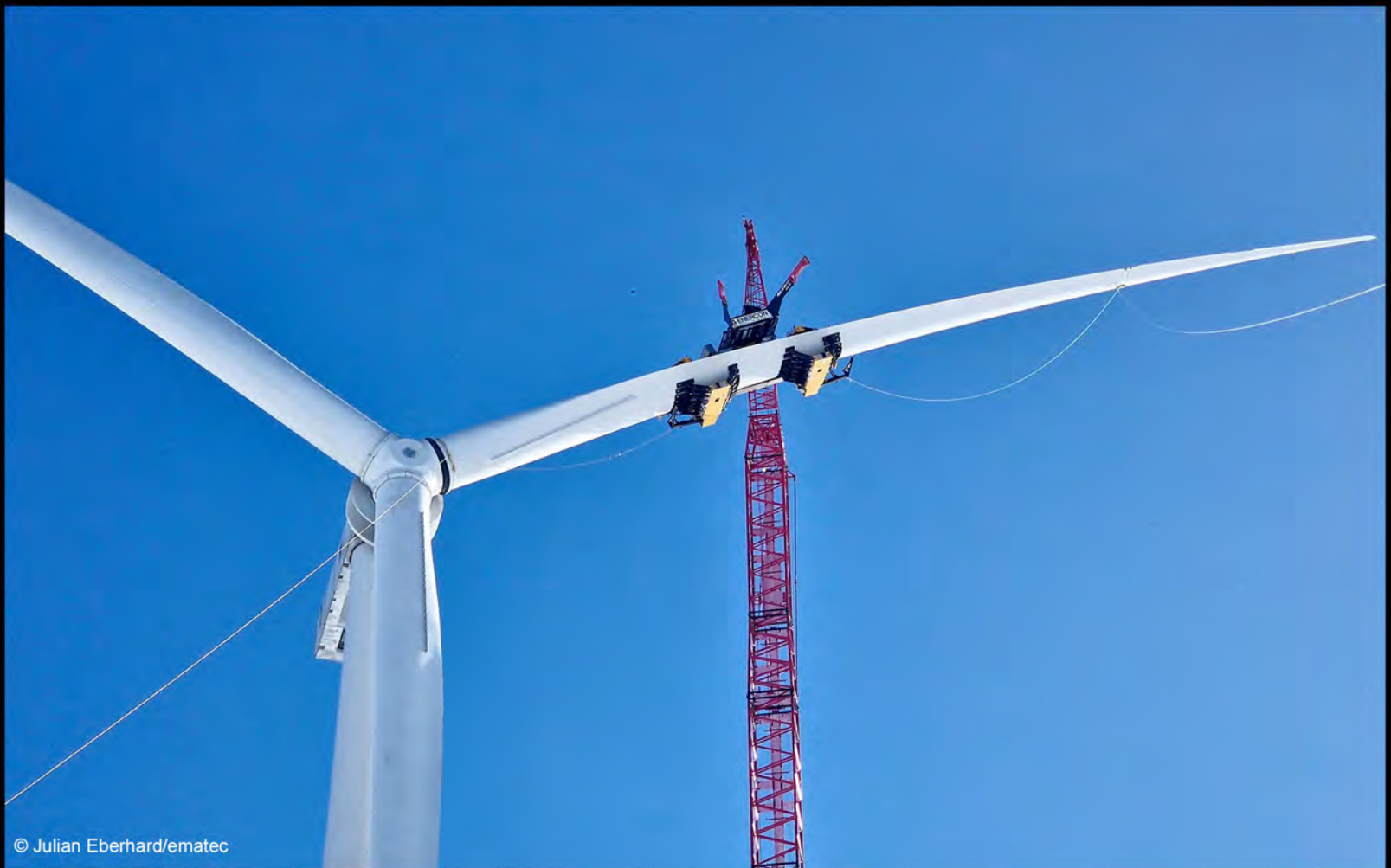
The RBC-D50 rotor blade clamp from ematec in Canada
